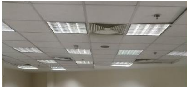
Figure 4: Existed Ceiling System
